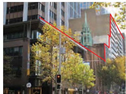
Figure 5.13 The top of the podium of the subject site complements the top of the facade of St Stephen's Uniting Church. The tower of the St Stephen's Uniting Church is visible above the podium. The building height increases to the north of St Stephen's Uniting Church along Macquarie Street.
