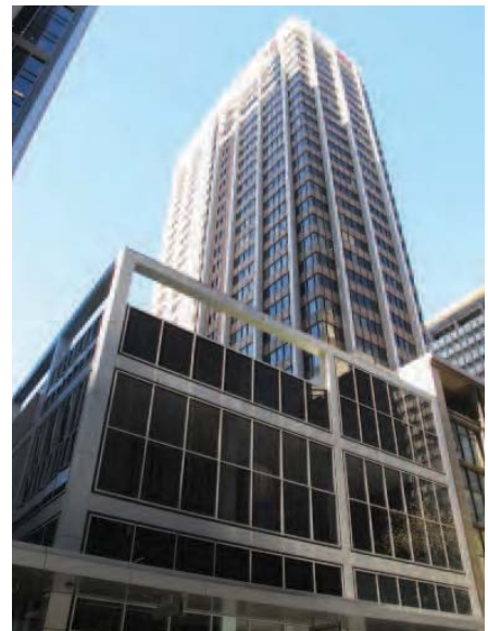
Figure 3.38 The tower of 60 Martin Place, as viewed from Phillip Street.
