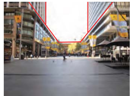
Figure 5.9 The current height of the podium complements the height of the RBA building podium and the Sydney Hospital facade. These frame the skyline at the eastern end of Martin Place. The setbacks of the towers of the subject building and the RBA building contribute to this.
