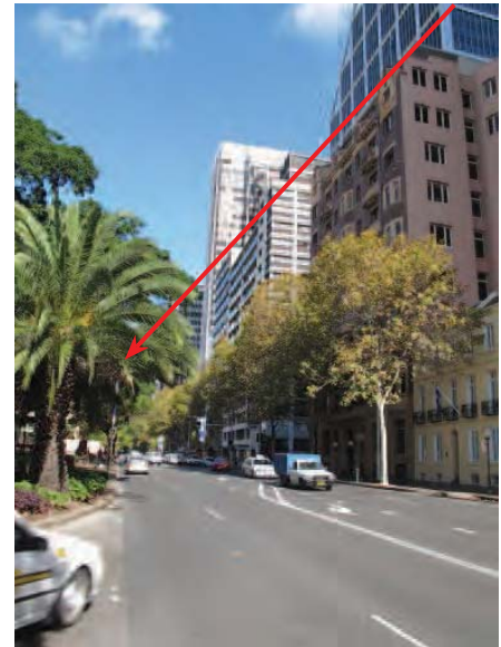
Figure 5.11 The tower of the subject building sits above the general building wall height along Macquarie Street. The eastern elevation of the building makes little contribution to the Macquarie Street wall.
